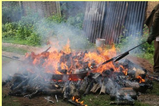
**Heating the iron tyre to about 800<sup>0</sup> C**
